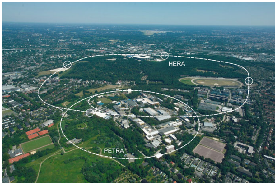
Fig. 8.11 HERA's intersecting electron/positron and proton rings. The detector in the straight sections is also shown
