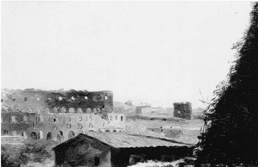
Figure 1. Pierre-Henri de Valenciennes (1750–1819). View of the Colosseum . Photo: C. Jean. Photo Credit: Réunion des Musées Nationaux/Art Resource, N.Y., Louvre, Paris, France
