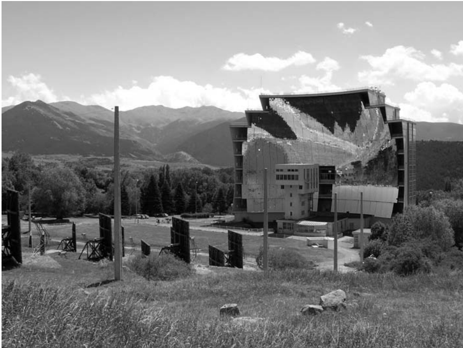
Fig. 15.15. The largest solar furnace at Odeillo. Several heliostats can be seen in the foreground. (Photo by Serge Chauvin.)
