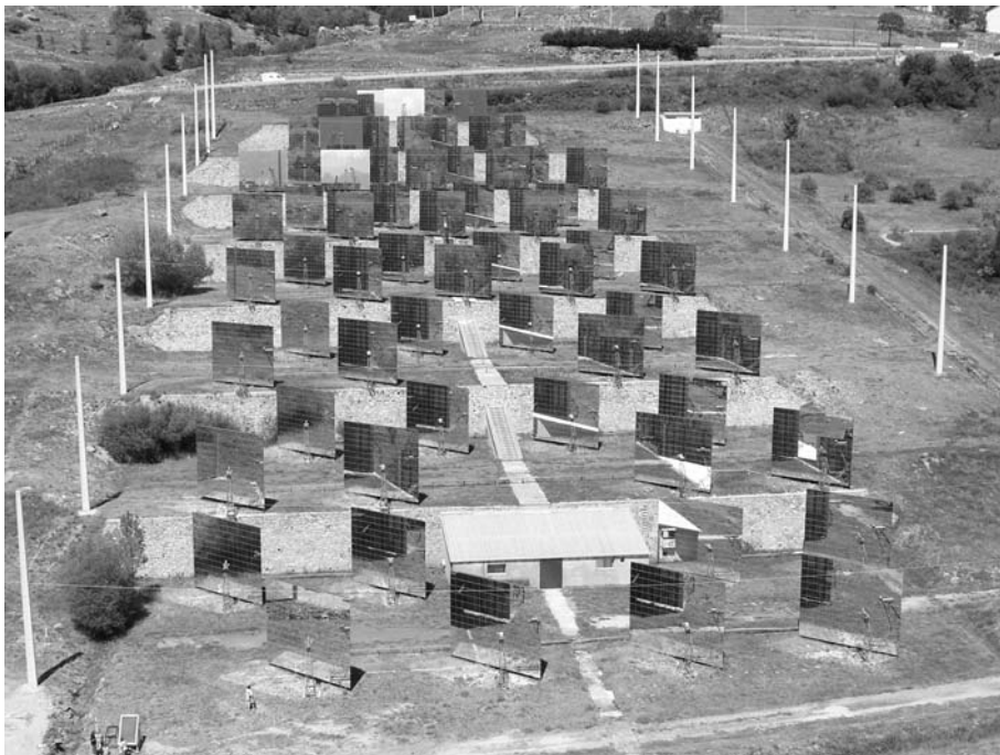
Fig. 15.16. Heliostats redirect the solar rays toward the primary parabolic mirror of Odeillo's solar furnace (photo by Serge Chauvin).
