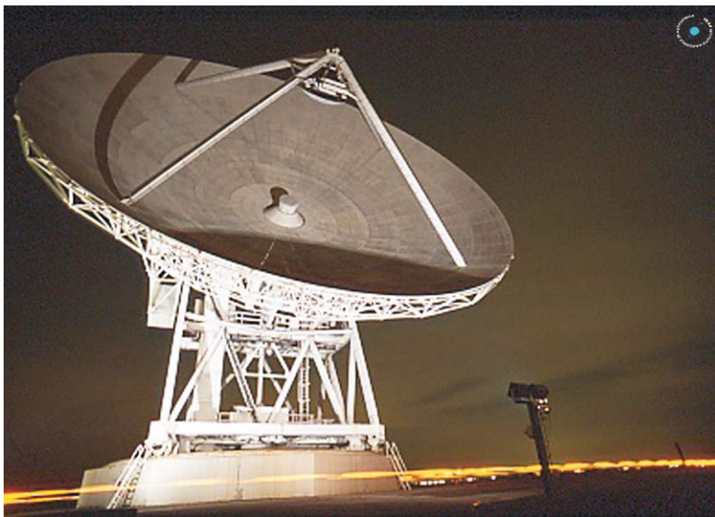
Fig. 5.6 The Medicina 32 m radiotelescope. The 32 m parabola is used both in single dish and for interferometric observations. The frequency coverage is between 1.4 and 22 GHz
