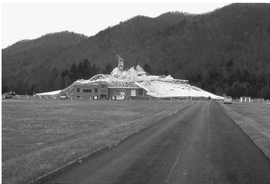
FIGURE 15.1. At 9:43 pm EST on Tuesday the 15th of November 1988, the 300-ft telescope in Green Bank collapsed. The collapse was due to the sudden failure of a key structural element—a large gusset plate in the box girder assembly that formed the main support for the antenna. This is a photograph of the 300-ft telescope taken on November 16, 1988 after the collapse. The loss of the 300-ft telescope resulted in the Green Bank Telescope project, Figure 15.2. (Photo Richard Porcas, courtesy of the NRAO/AUI.)
