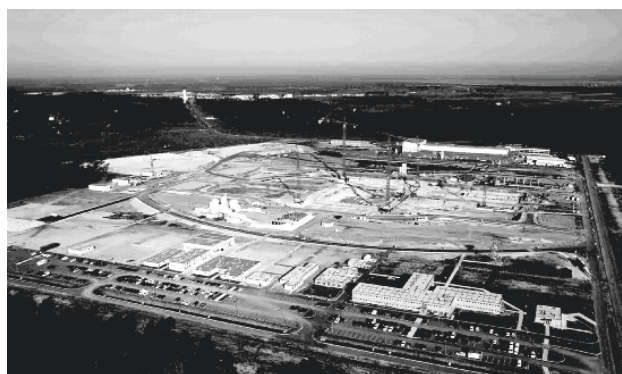
Fig. 5.12. Aerial view of the construction site
