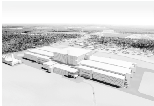
Fig. 5.9. Artist view of the future LMJ facility
