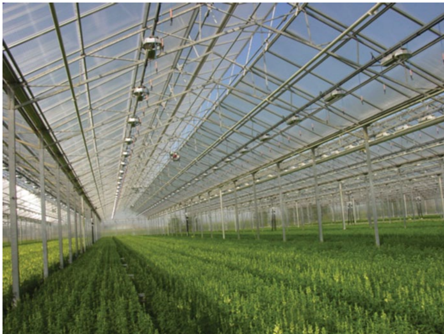
Fig. 11.10 Example interior of a modern-day greenhouse range in Canada, glazed with rigid Exolite for growing cut snapdragons, Antirrhinum majus . (Photo credit: Neil Anderson)
