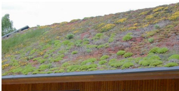
Fig. 12.8 Roof garden containing a range of Sedum pp. (Photograph courtesy of A. Bettin)
