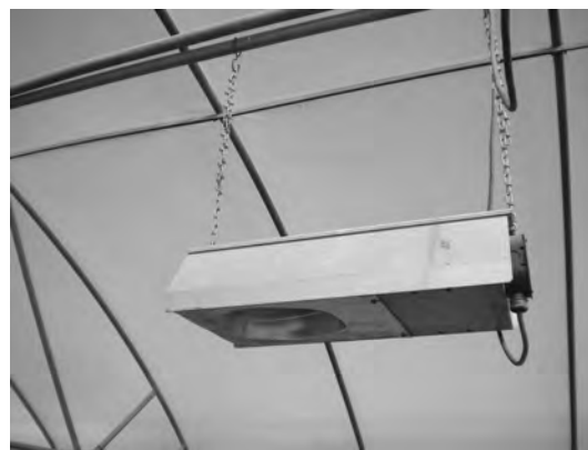
Fig. 8.1. A high pressure discharge luminaire for supplemental greenhouse lighting.
