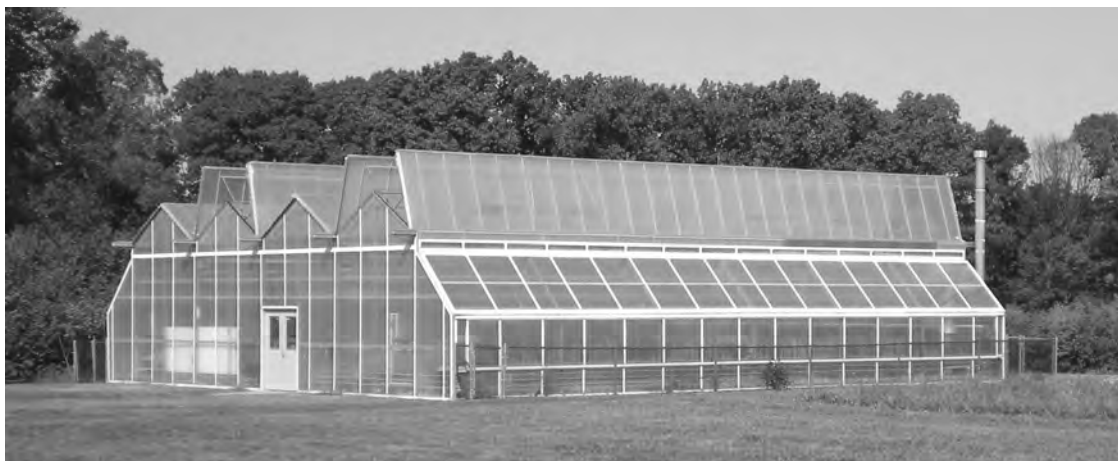
Fig. 11.3. Natural ventilation of an open roof greenhouse.
