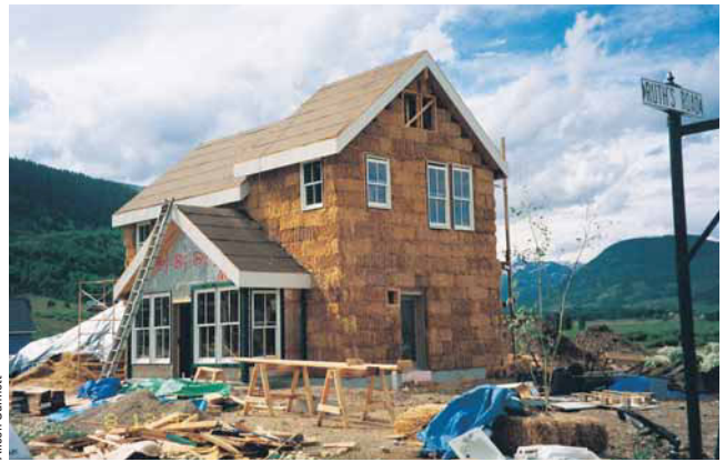
Photo 9 Energy efficient straw bale house in Crested Butte, Colorado (USA) during construction
