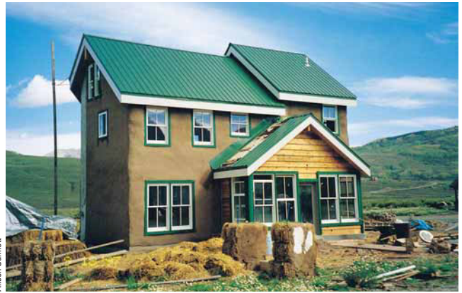
Photo 10 Completed energy efficient straw bale house in Crested Butte, Colorado (USA)
