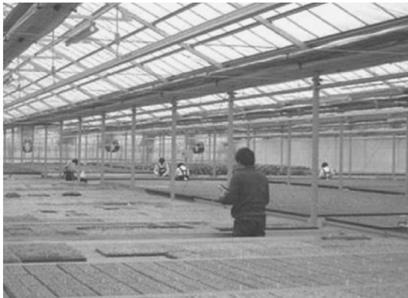
Figure 5. A conventional greenhouse covered with glass sheets. In order to use solar light that is free of charge, many kinds of environmental control equipment often need to be installed for ventilation, heating, heat conservation (thermal screen), shading, watering, etc. Much fuel or other kinds of energy are also necessary. In order to lessen the rapid changes with time in air temperature and relative humidity, a tall greenhouse (6-10 m high) with large air mass is needed for growing short transplants with only about 0.1-0.2 m high, which is space inefficient and costly.
