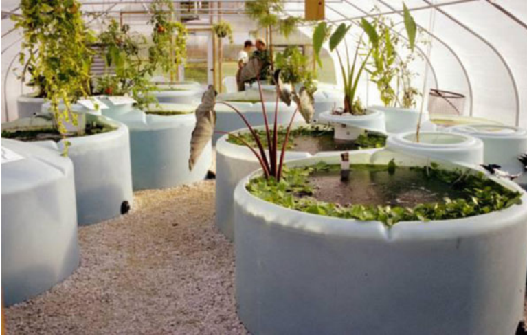
Figure 5. Eco-machine treating brewery waste (Image: John Todd).
