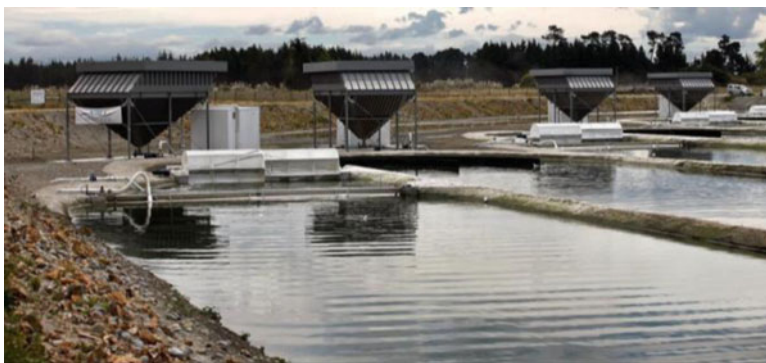
Figure 5. HRAP + C system (5 ha) operating in Christchurch, New Zealand.
