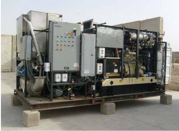
Fig. 4 TGER after retrofit
