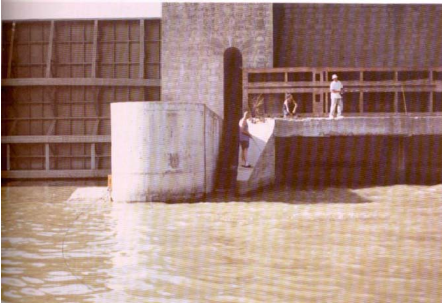
Fig. 26.5 View of the fish ladder at Alcalá dam, as can be seen by comparison with the people shown, the dimensions of the ladder being completely inadequate for sturgeons. Figure taken from the magazine Azotea , vol. (13–14) from the town hall of Coria del Río (Sevilla province)
