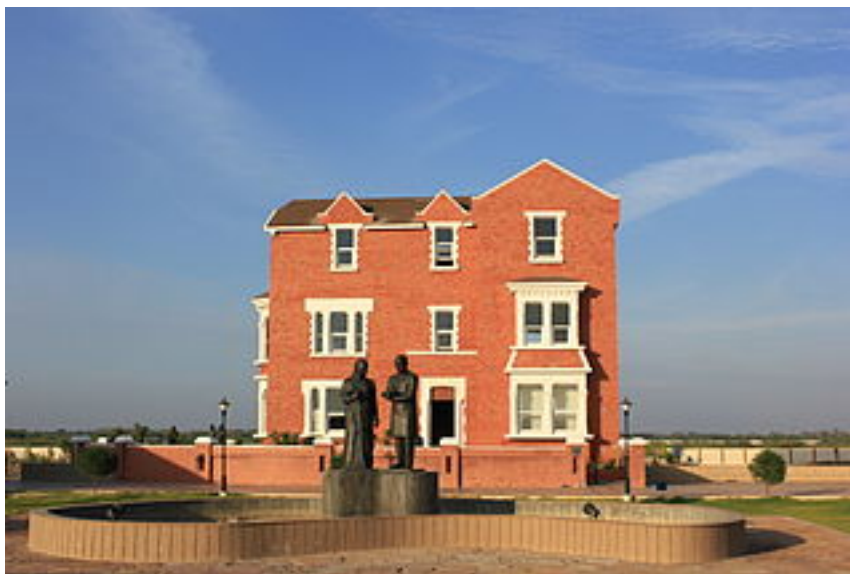
Fig: Varma House, replica of the India House of London used by shyamaji Krishna Varma for revolutionary activities in Gujarat, India
